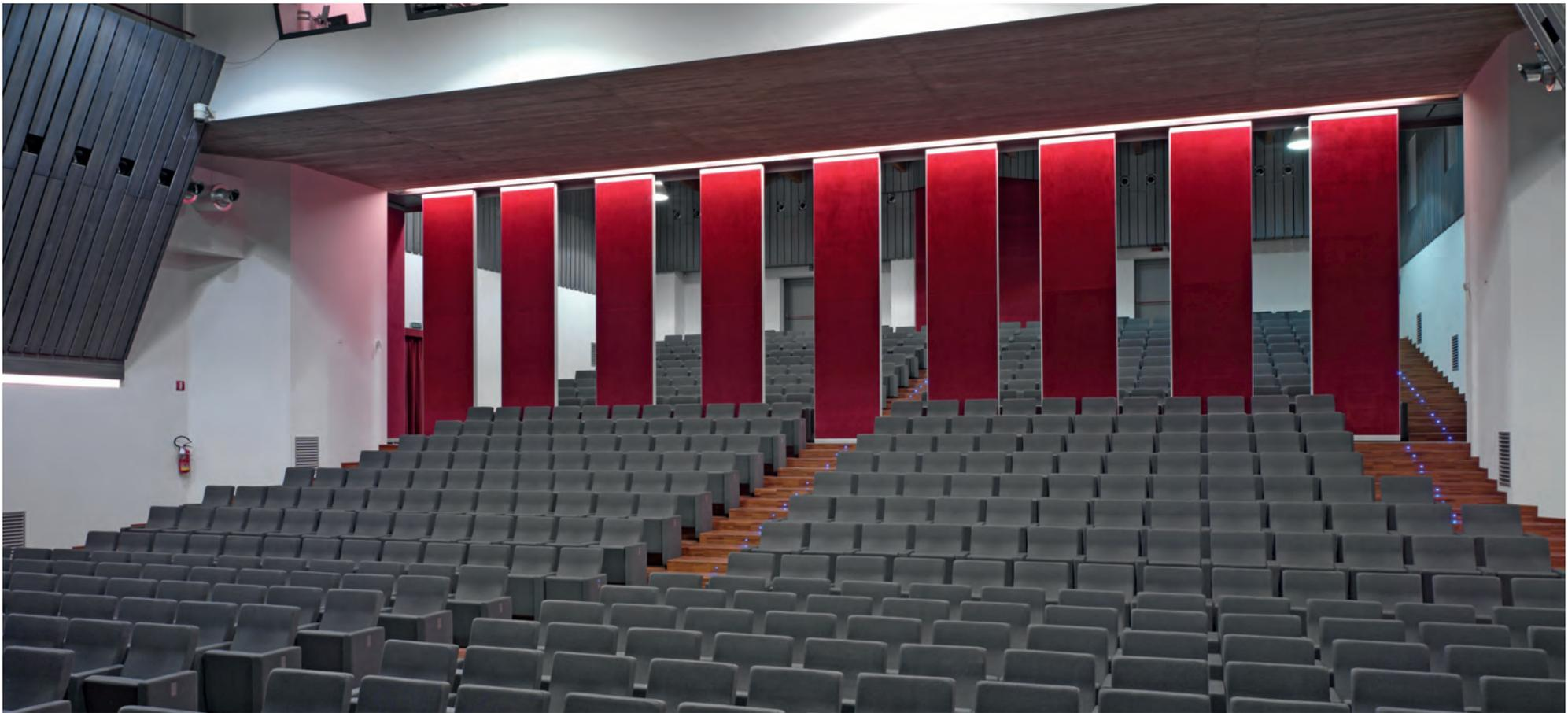
Since 1980 the company started with the production of movable partitions, composed by independent elements which slide by ball bearing trolleys in a track fixed only to the ceiling. The easy way of using and the infinite possibility to split big spaces have decreed the big success of the product.
