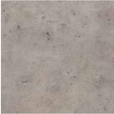
Exposed Concrete AROSEC30
